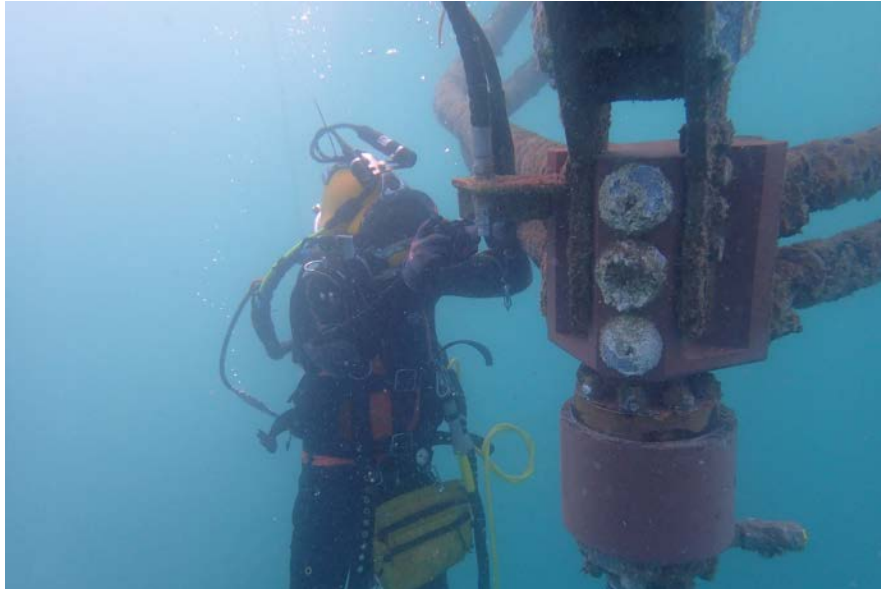
Diver inspecting Unit #2 stab connection after Unit release
