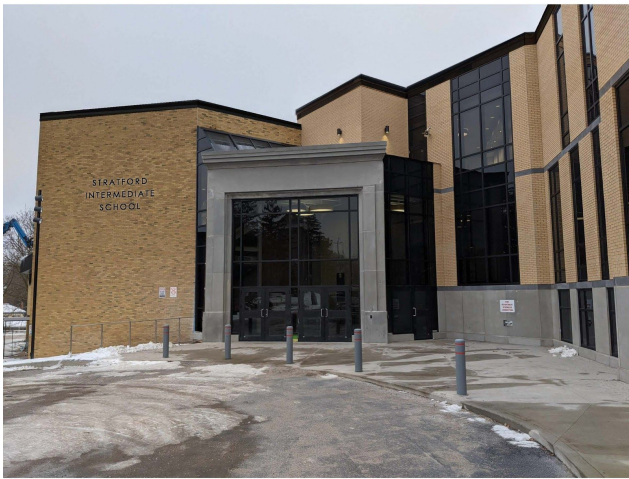
Photo 1: New main entrance
